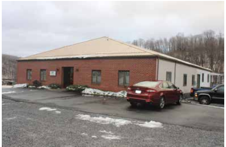
AT HOME IN BEDFORD COUNTY; Cell-Con is located along Route 220 South in Bedford Valley.
